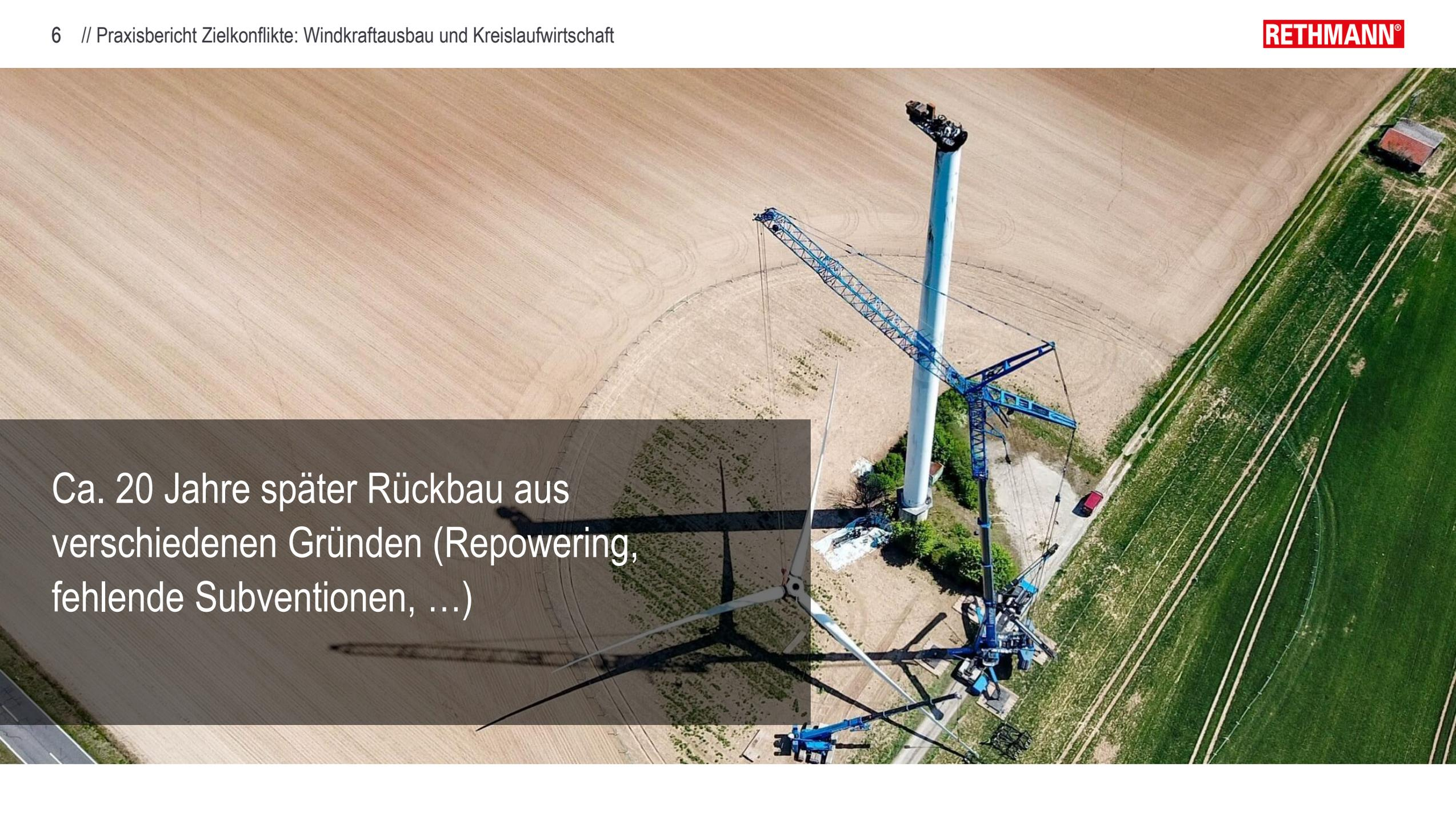
An aerial photograph showing the dismantling of a wind turbine tower. A large blue lattice crane is positioned on a dirt road, lifting a section of the white tower. The tower section is suspended in the air. The surrounding area consists of a large brown field and a green field with a red barn in the distance. A red car is parked on the road near the crane. The wind turbine's nacelle and blades are visible in the lower part of the frame.
